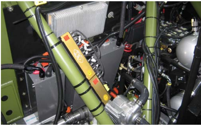
Figure 6 - FED BRAVO Rear Compartment Electronics
